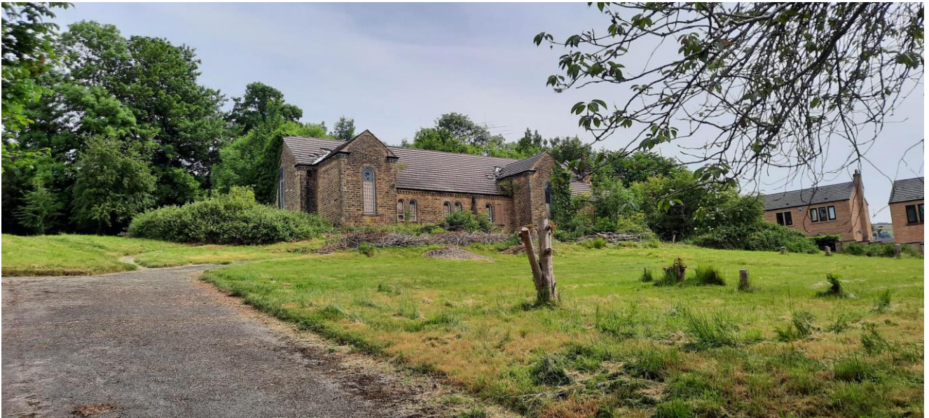
View of site including the former Church of Christ the King from the site entrance on Bradford Road
